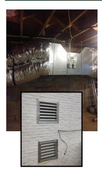
"One call to BPE, and I was able to get permit approval," says Sam. BPE determined that the salon required approximately 900 cfm of air exchange. Consequently, he recommended the BPE-XE-MIR-1000 energy recovery ventilator (ERV) for providing enough outdoor air. The unit was set up in the cellar.
